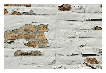
Paint and stain may present aesthetically similar appearances on concrete and similar surfaces. However, that correlation is only skin deep. The fundamental difference in how they color a surface makes stain the superior choice for concrete and masonry surfaces within communities.
